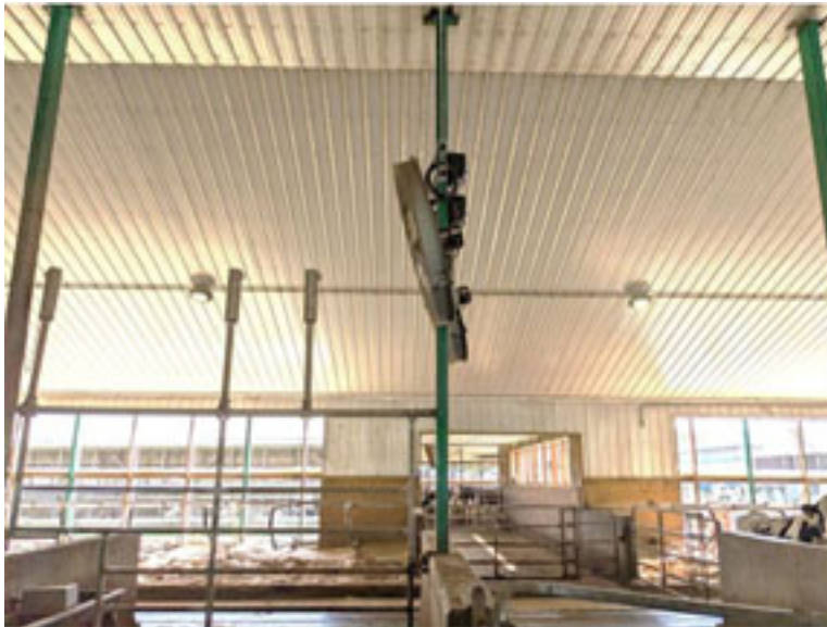
Figure 9. Fan showing current installed angle. Effectiveness of Fans for Heat Stress Abatement on Lactating Dairy Cows in NNY project, NNYADP, 2023.
