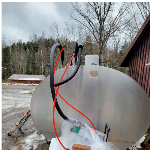
Figure 2: Left: the larger DIY chiller connected to the cooling plates on a 1500-gallon insulated dairy tank. These lines typically pump refrigerant through the cooling plate but glycol can be pumped through the plates. Right: the smaller DIY chiller connected to a cooling plate submerged into an open top tank.
